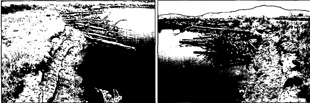
Figure 5-7. Examples of engineered log jams on the Sprague River. Upstream (left) and downstream (right) views of two structures illustrate the bank protection and aquatic habitat creation benefits of the structures. Willow cuttings planted in the soil lifts will provide additional bank stability and riparian habitat in the future.
