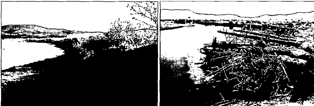
Figure 5-5. An example river corridor condition in the downstream portion of the assessment reach (left). A woody debris jam constructed on the Sprague River provides bank protection and diverse habitat for fish and wildlife (right).
