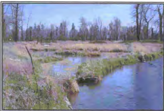
Figure 6.2: Finger bars are effective for narrowing over-widened channels. These structures require minimal fill material and create off-channel pond habitats. Off-channel habitats may benefit juvenile shortnose and Lost River suckers out-migrating from Anderson Spring Creek. The ponds also benefit waterfowl.
