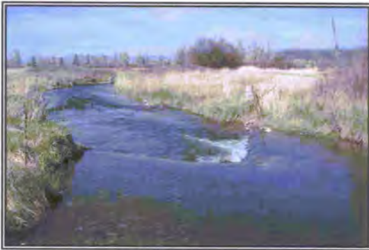
Figure 6.1: A log weir provides fish habitat and directs the thalweg towards the center of the channel, reducing lateral bank erosion and sediment contributions.
