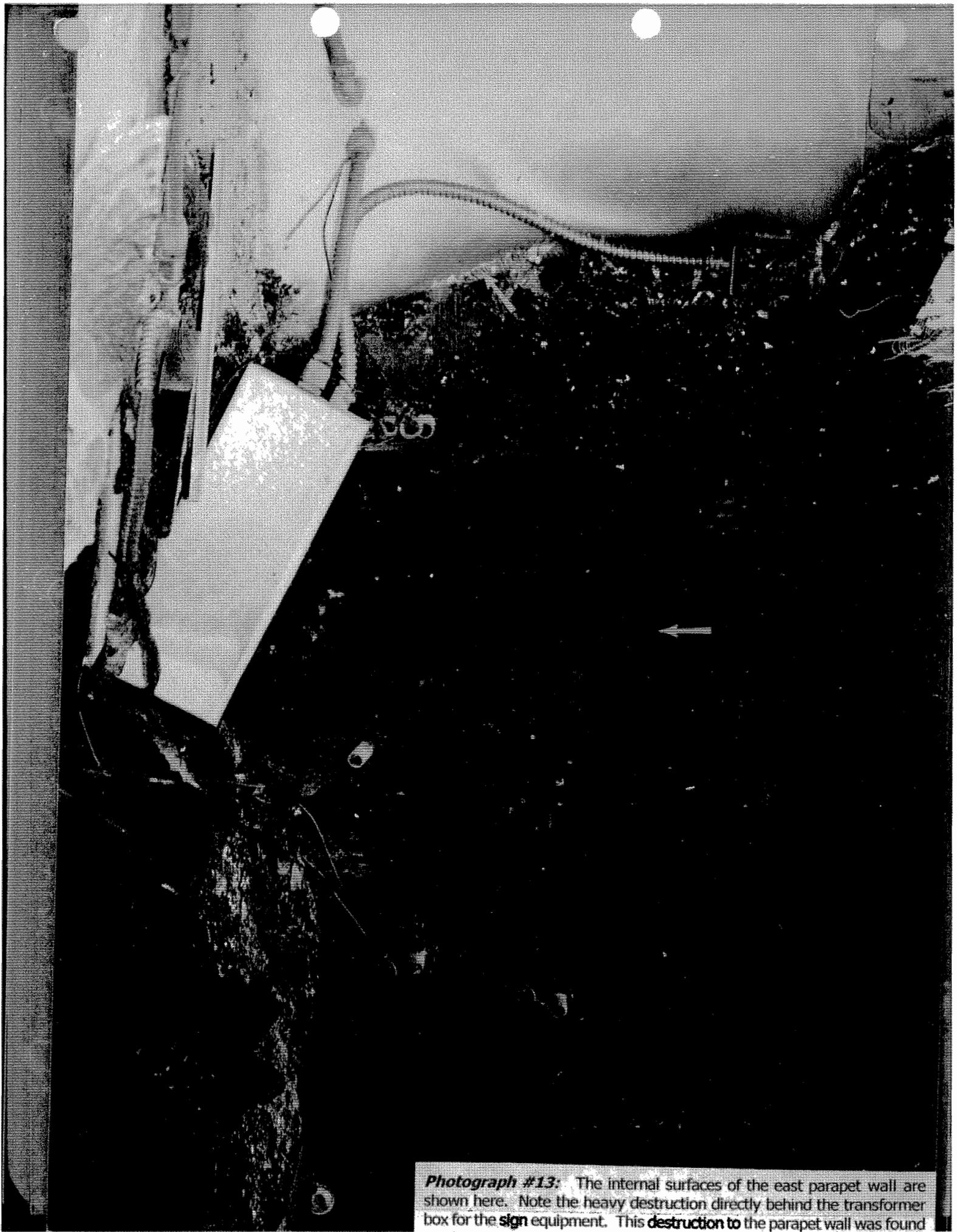
**Photograph #13:** The internal surfaces of the east parapet wall are shown here. Note the heavy destruction directly behind the transformer box for the **sign** equipment. This **destruction to** the parapet wall was found
